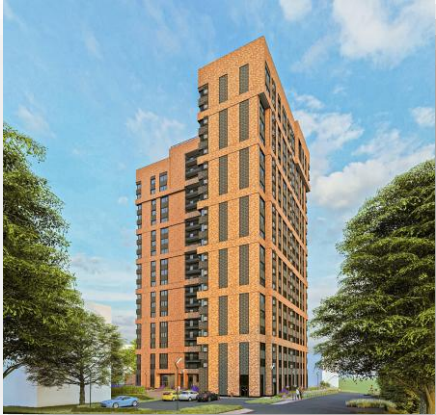
Renovation, Mozhaisky, Gorbunova str.
