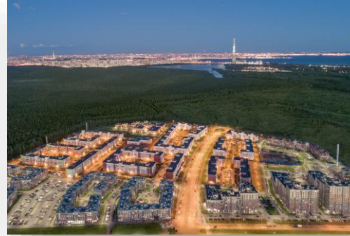
Yuntolovo Residential Complex, St. Petersburg
